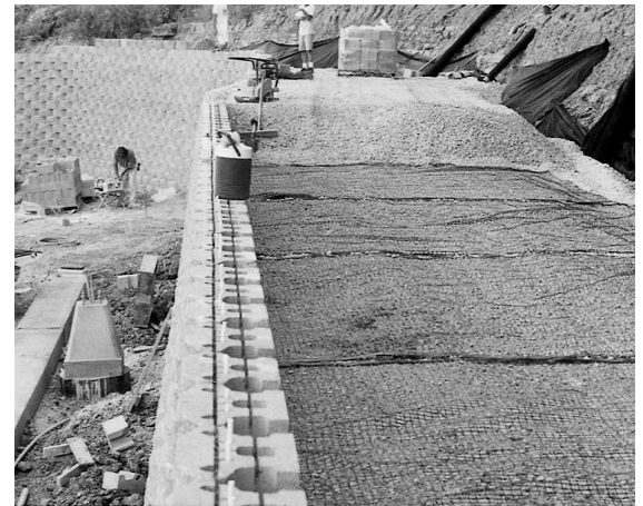
Figure 1 Miragrid 5XT in SRW
