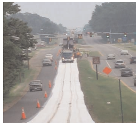
Above: 2” of HMA being installed. Below: Installation of TruPave® Engineered Paving Mat
