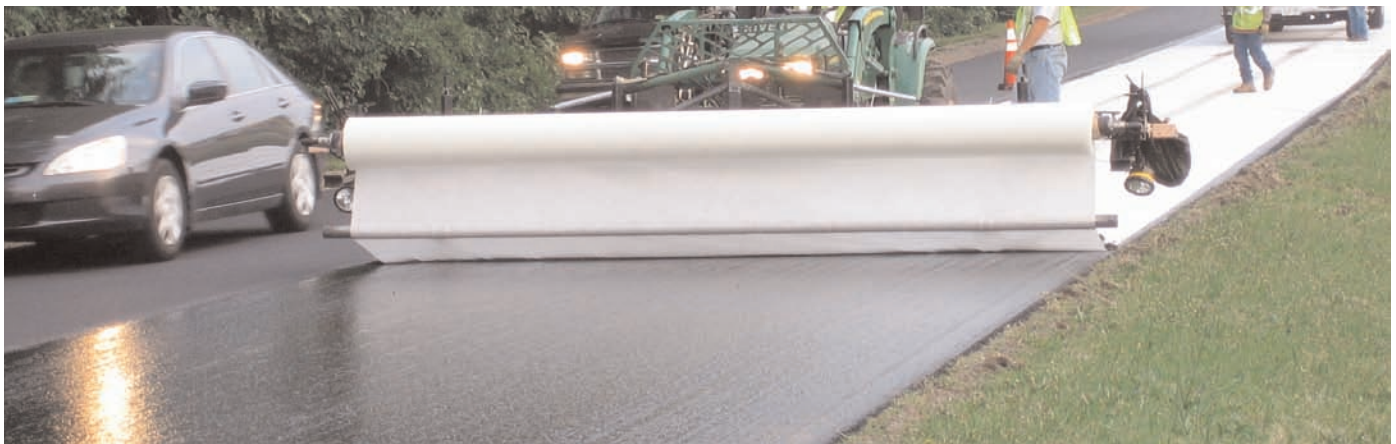
Below: Installing with laydown tractor.
