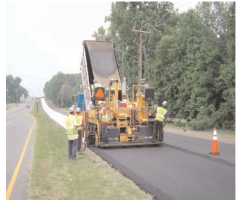
Above: 2” of HMA being installed. Below: Installation of TruPave® Engineered Paving Mat
