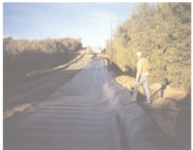
Mirafi® HP570 is rolled out over the subgrade. Mirafi® HP570 serves two functions: to reinforce and separate.
