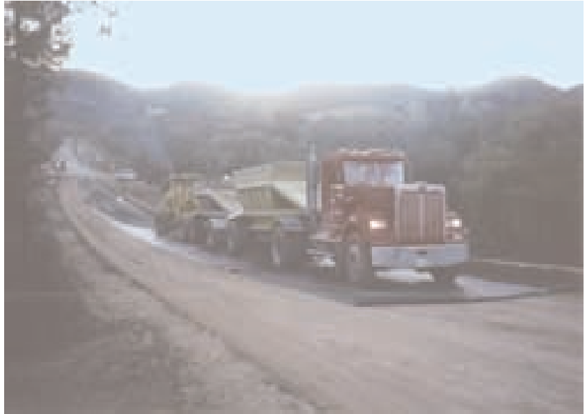
Fill was dumped and levelled over the fabric.
