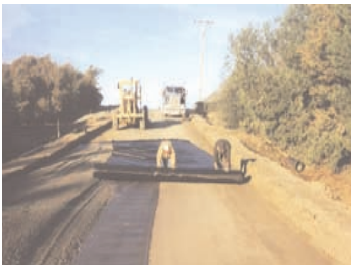
Mirafi® HP570 is rolled out over the subgrade. Mirafi® HP570 serves two functions: to reinforce and separate.
