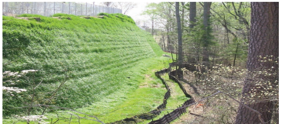
Reinforced slope outside of the Gwinnett Braves Stadium.
