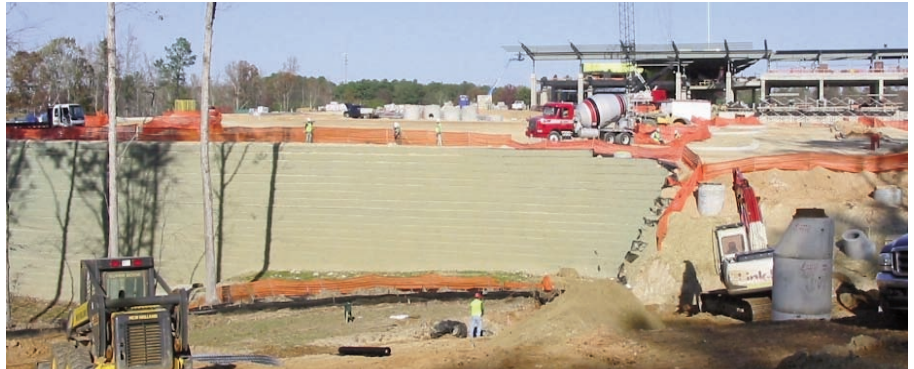
Construction of the existing wall into a reinforced slope.
