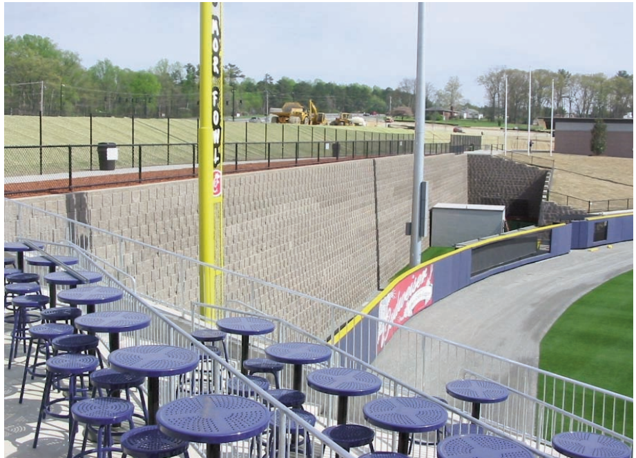
Completed retaining wall at the Gwinnett Braves Stadium.
