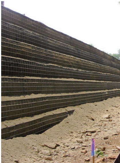
Reinforced slope outside of the Gwinnett Braves Stadium.
