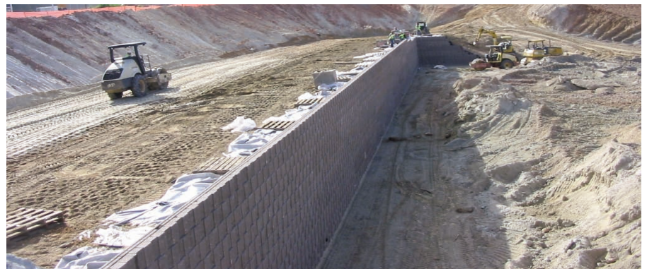
Construction of the outfield retaining wall.
