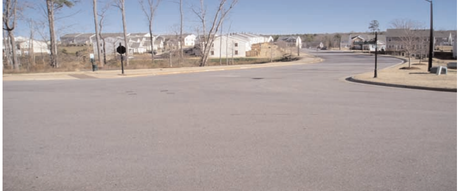
HP reinforced intersection at Country Trail and Marvino Lane.
