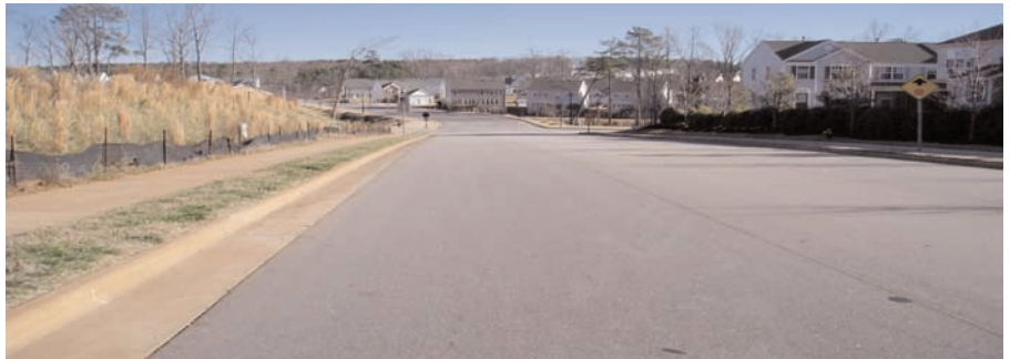
View down Country Trail reinforced with Mirafi® HP370.
