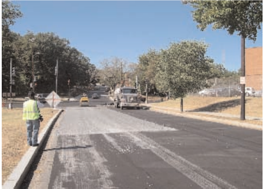
Chip seal over Mirafi® MPV500 paving fabric.
