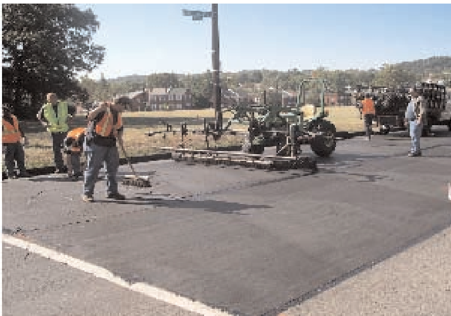
Installation of the fabric.
