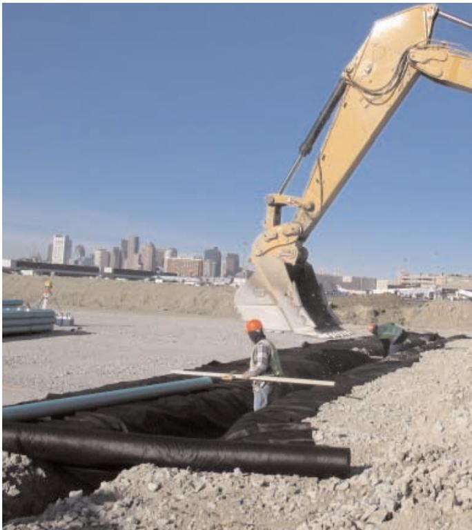
Constructing taxiway edge drain with Mirafi® 140N drainage fabric.
