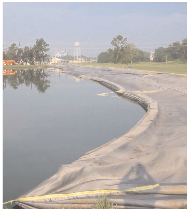
Deployment of approximately 75,000sy of Mirafi® HP770PET.
