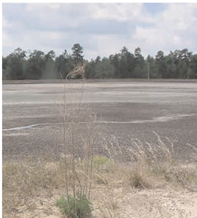
Pre-construction picture of lagoon.
