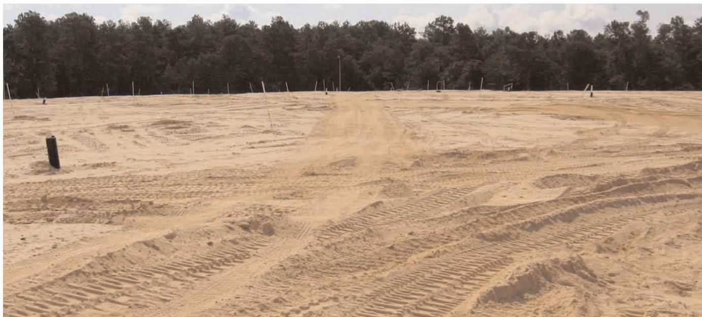
Nearly completed cap without vegetation.
