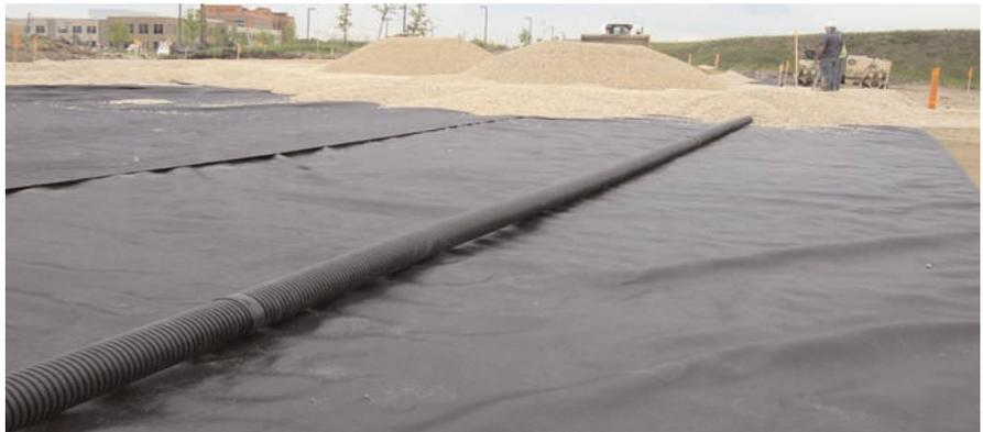
Drainage pipes laid during aggregate placement.
