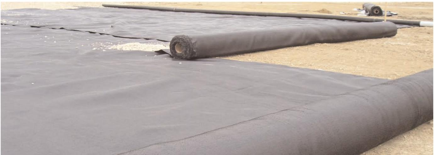
Mirafi® HP570 being rolled out with an 18” overlap.
