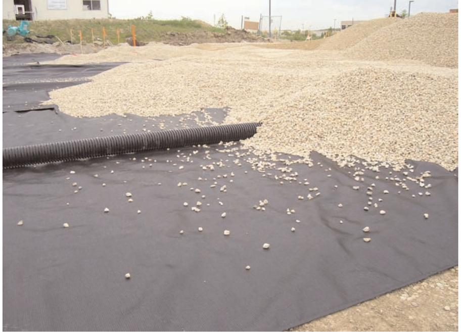
Open graded stone being placed over the drain tiles.
