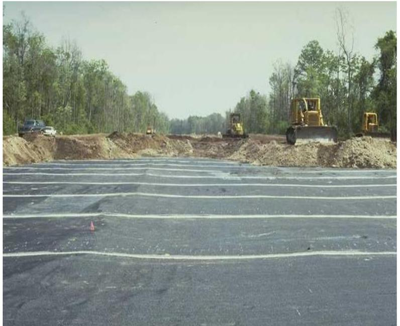
Figure 1. Seamed Geotextile Panel
