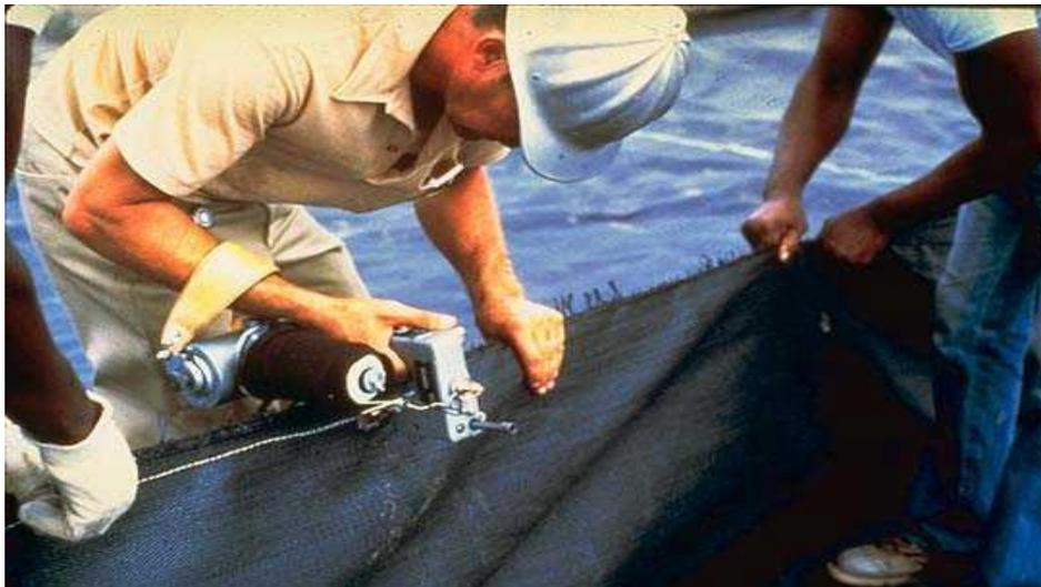
a) a handheld sewing machine, and b) double-needle stitch sewing machine. Figure 3 illustrates the field sewing of geotextiles using the hand-held machine. Figure 4 illustrates factory seaming using a double-needle stitch sewing machine.
