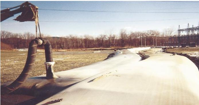
Figure 1: Geotubes in spoils area. Each tube contained 500-600 CY of spoils.
