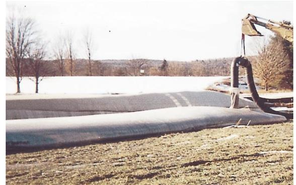
Figure 2: Geotubes being filled with dredged material from the plant's intake area.
