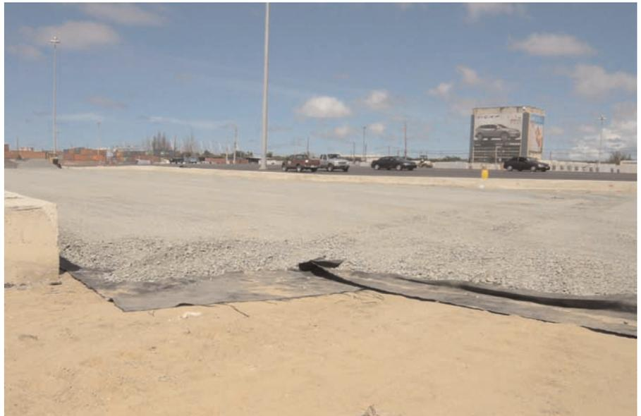
The use of two high strength geosynthetic layers allowed for the required pavement strength while minimizing the overall thickness.
