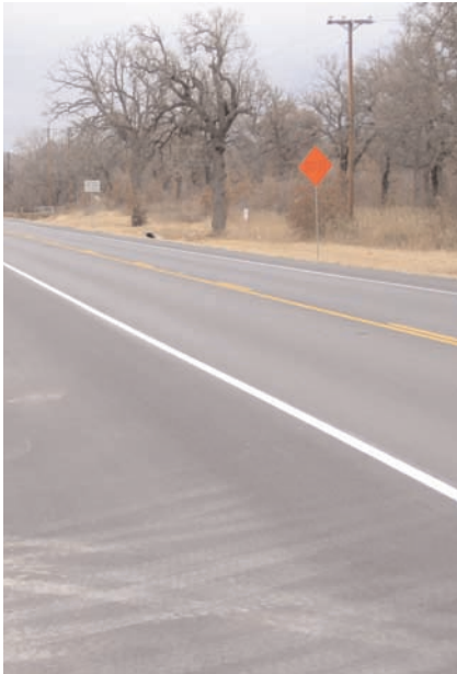
Finished construction of Mirafi® MPV500 and asphalt overlay.
