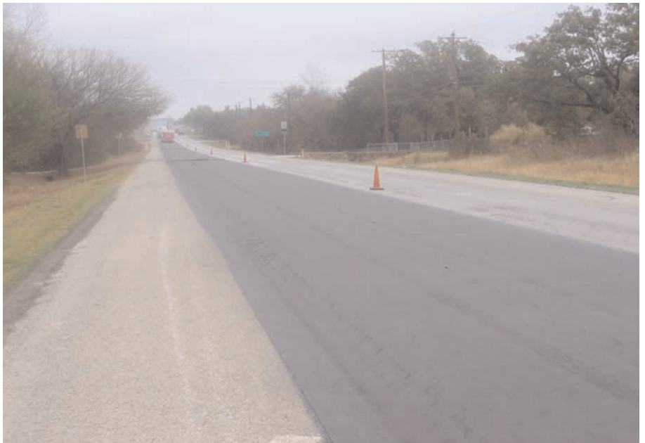
Finished installation of Mirafi® MPV500.
