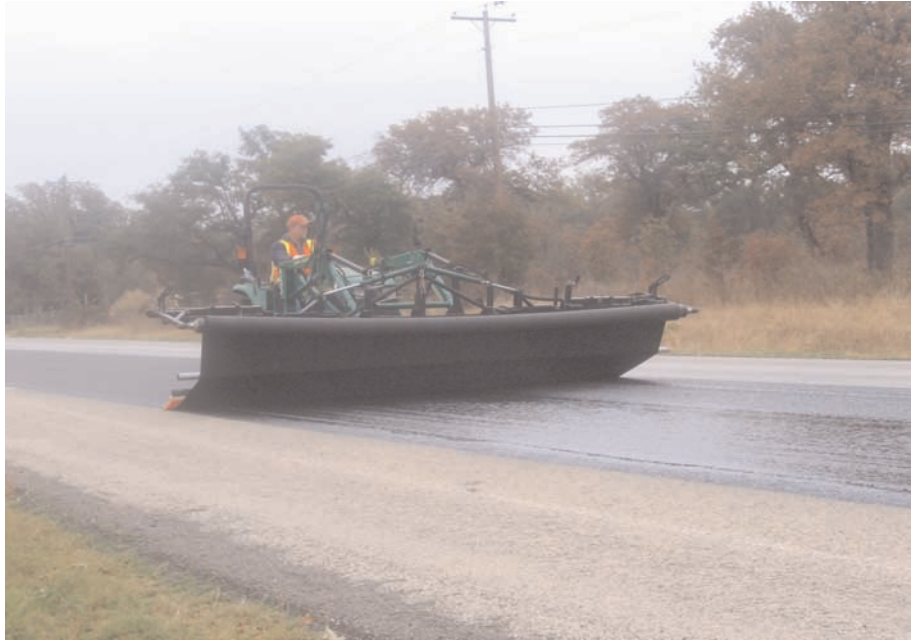
Installation of Mirafi® MPV500.
