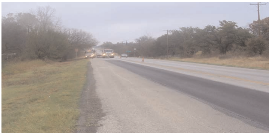
Roadway condition prior to installation of Mirafi® MPV500.
