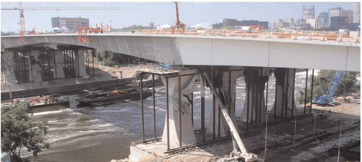
I-35 bridge over river.
