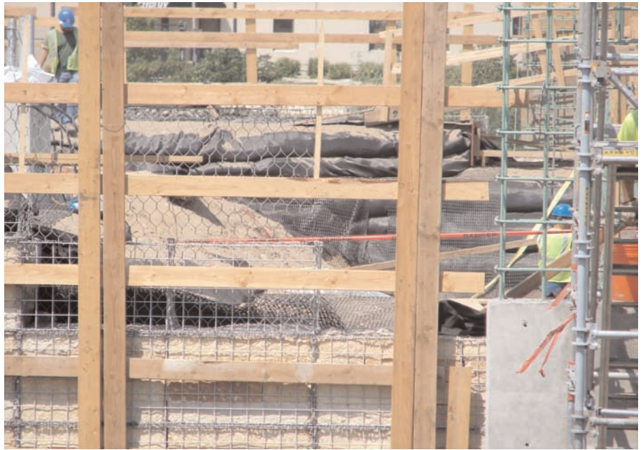
Gabion Wall at bridge abutment. Fabric wrapped wall in background.
