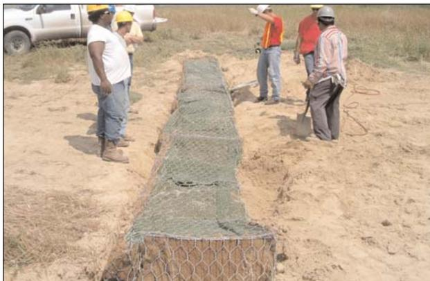
Workers install Miramesh™ GR lined gabion baskets in trench across channel.
