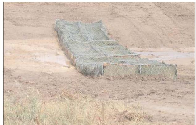
The baskets effectively dam water, allowing sediment to drop out upstream.
