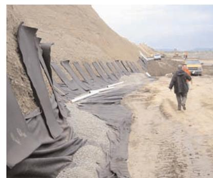
filter fabric easily rolled out and held up well to the placement of the 3/4 minus drain rock. The owner and contractor were pleased with the outcome of the project.
