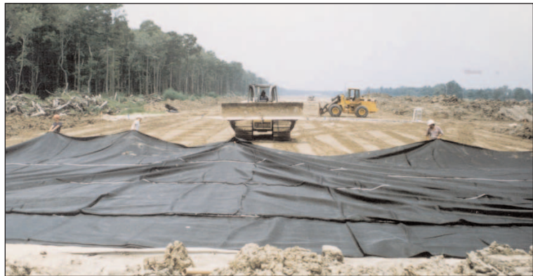
In this test, both woven polypropylene and woven polyester geotextiles are compared to geogrids.
