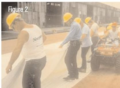
The deployment of the two geotextile sheets took place on two weekends when both runway closures and midday high tides coincided. The 2.1m (7 ft) Tidal range at the airport provided the barges with sufficient draft at high water to come within 15 meters (50 feet) of the shoreline. The leading edge of the geotextile sheet was pulled to shore and secured (Figure 3).
