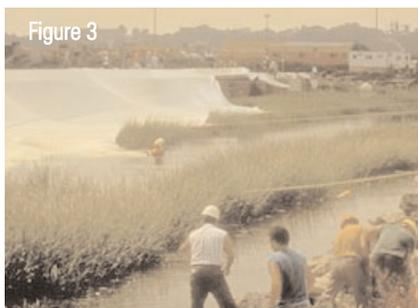
The barge assembly was then slowly pulled from shore with the geotextile unfurling into the water and progressively sinking onto the bay bottom, where it was secured with sandbags. In the area immediately behind the runway, which is subject to severe blast winds from jet aircraft,
