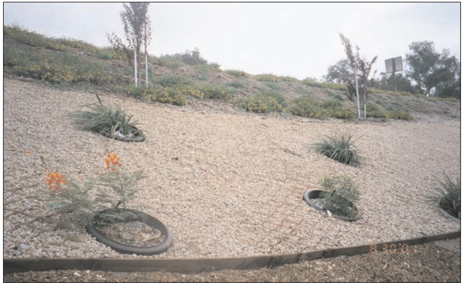
Microweb® is easily installed with J-hook stakes.
