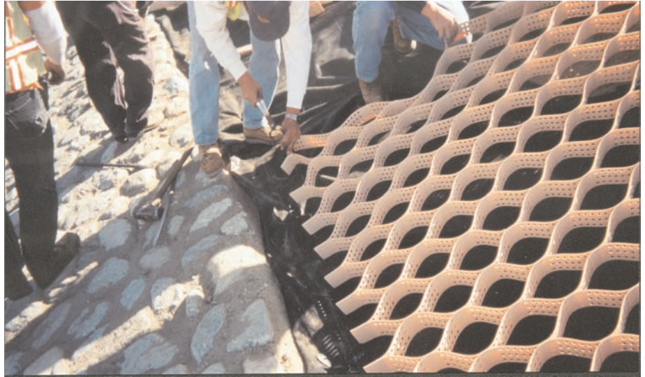
Microweb® is easily installed with J-hook stakes.
