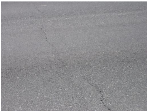
Figure 2: Application rate - 0.25 gal/sy
