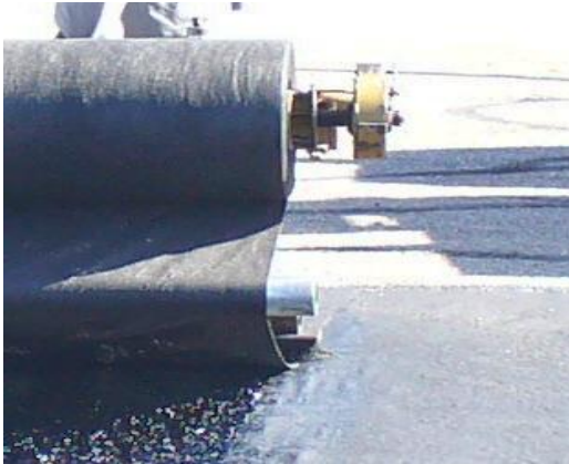
Figure 7: Longitudinal overlap
