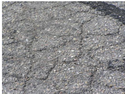
Figure 3: Application rate - .33 gal/sy
