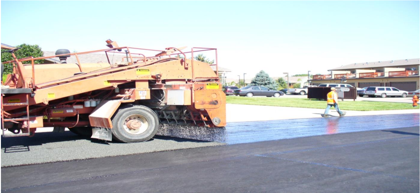
Figure 12: Chip sealing over paving fabric
