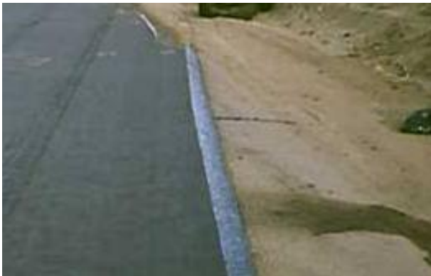
Figure 4: Tack coat beyond fabric
