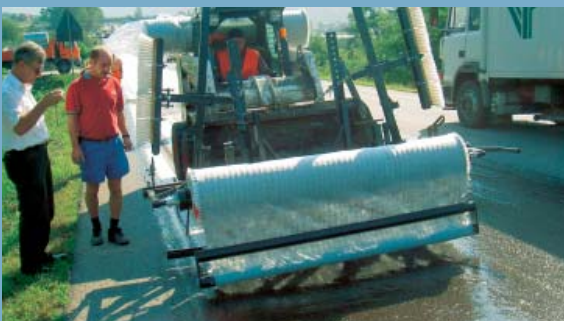
Geosynthetic installation with TenCate laying equipment.
