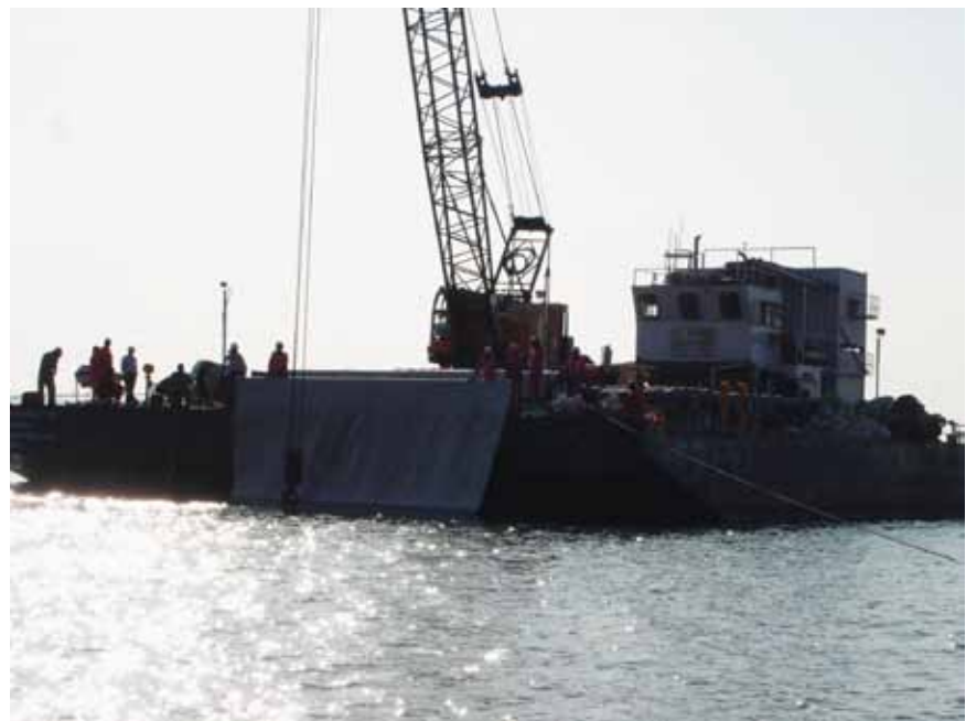
Installation of Polyfelt® TS009 nonwoven geotextile by using a floating barge
