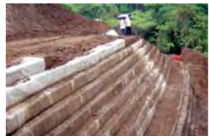
Slope repair works in progress
