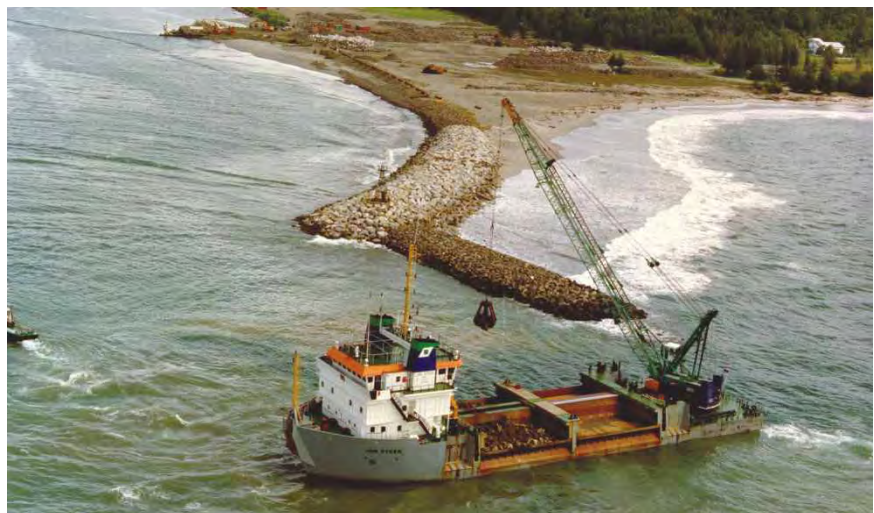
Construction of the breakwater
