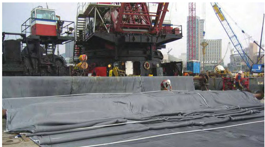
Preparation of the Mirafi® HP770 prior to development
