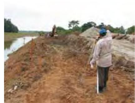
Setting alignment prior to Geobags installation.
