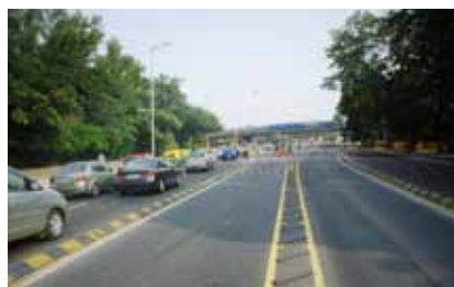
Overview of the BRT after construction.
