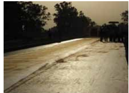
Installed Polyfelt® PGM 14 on the existing pavement.
