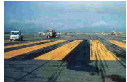
Figure 1: Runway prior to maintenance works
