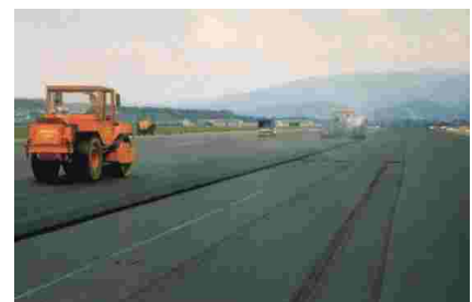
Figure 4: Installation and compacting of the asphalt concrete overlay
