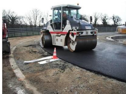
Figure 7. Pouring asphalt concrete on top of the sensor enabled geotextile strips (left) and compaction (right)
