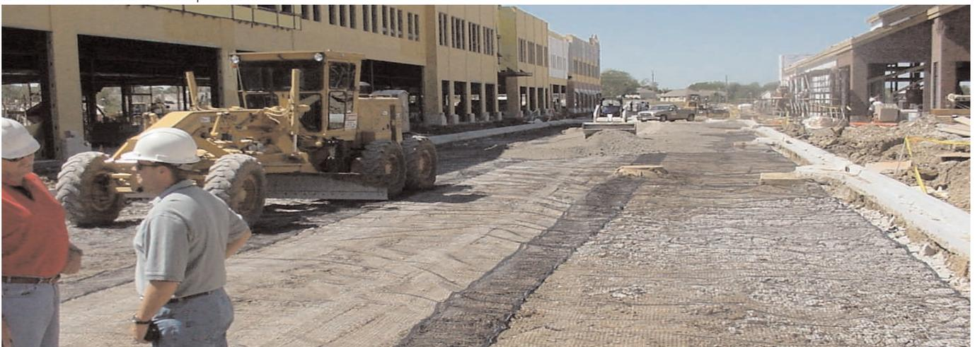
By installing Mirafi® BXG11 geogrid before the initial asphalt layer, construction traffic can use the road without damaging the pavement. After site construction was completed, no repairs to the road were necessary and the final asphalt leveling course was installed.
