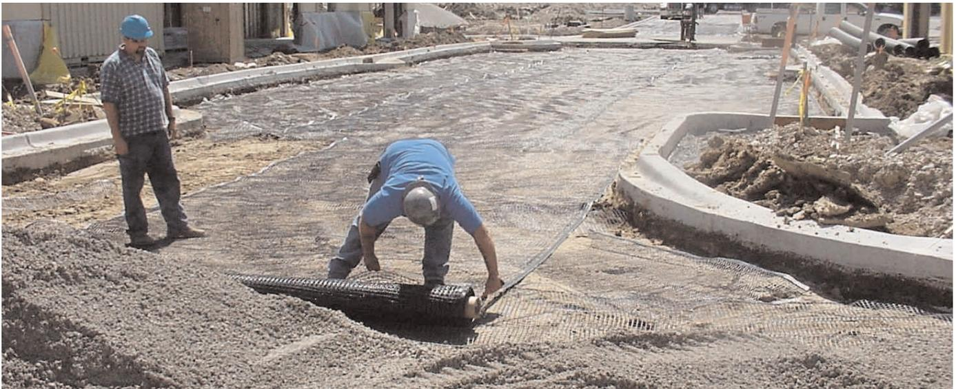
Mirafi® BXG11 geogrid prevented rutting and damage to the pavement, allowing the contractor to install the final asphalt layer while saving money and time.
