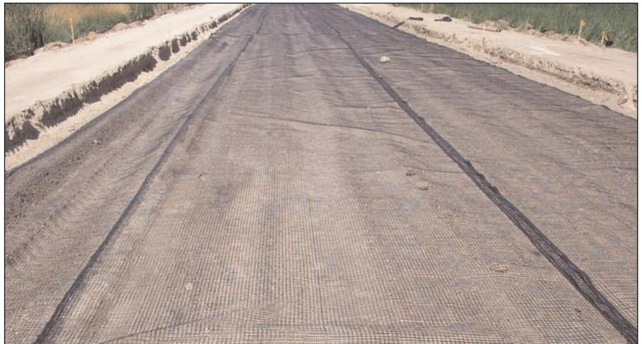
Mirafi® HP is used to separate soft subgrades from the base course, while providing the same high strength at low strains as geogrids.
