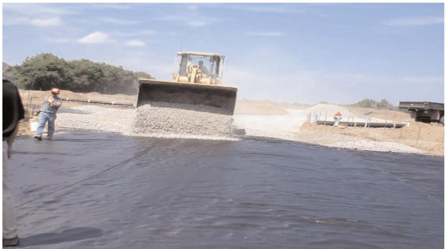
Mirafi® BXG11 geogrid is rolled onto the subgrade, then crushed concrete is placed on top.
