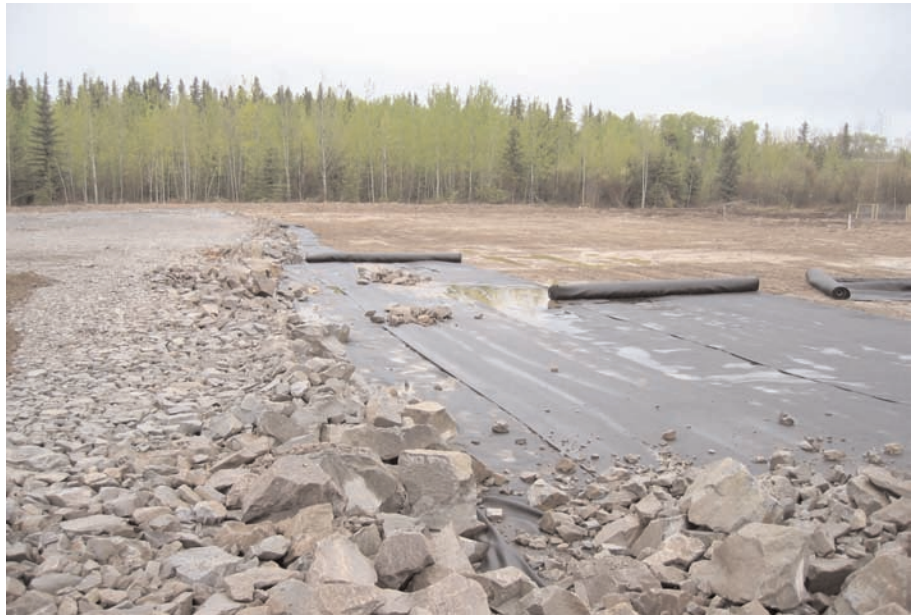
Blast rock and high permeability of Mirafi® HP570.
