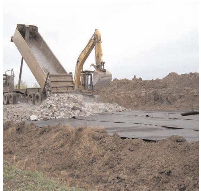
Blast rock placement and grading.
