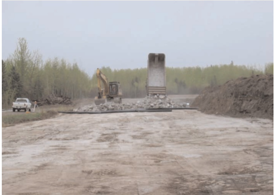
Proof rolled subgrade and rock placement.
