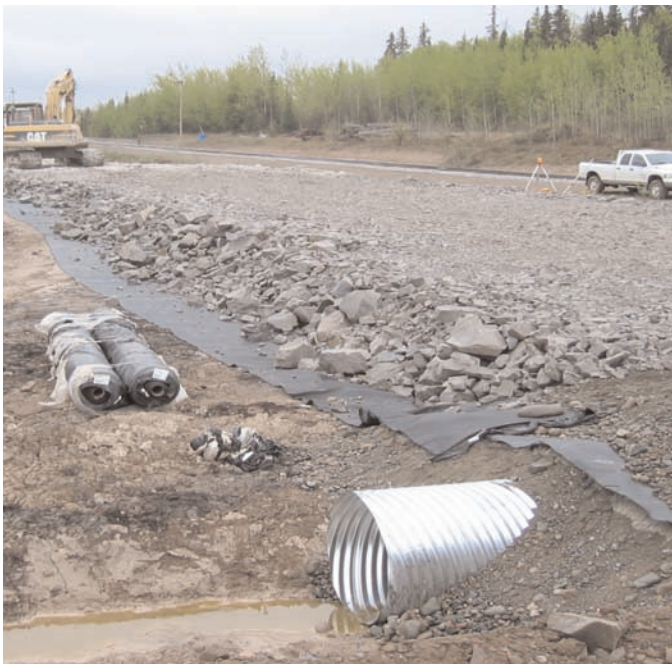
Completed road and yard area.
