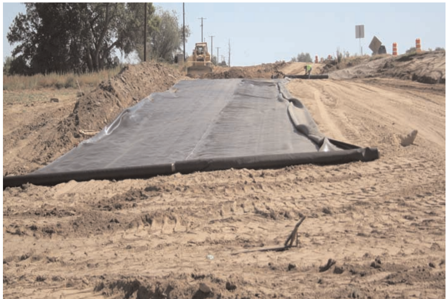
Installation of Mirafi® HP570.
