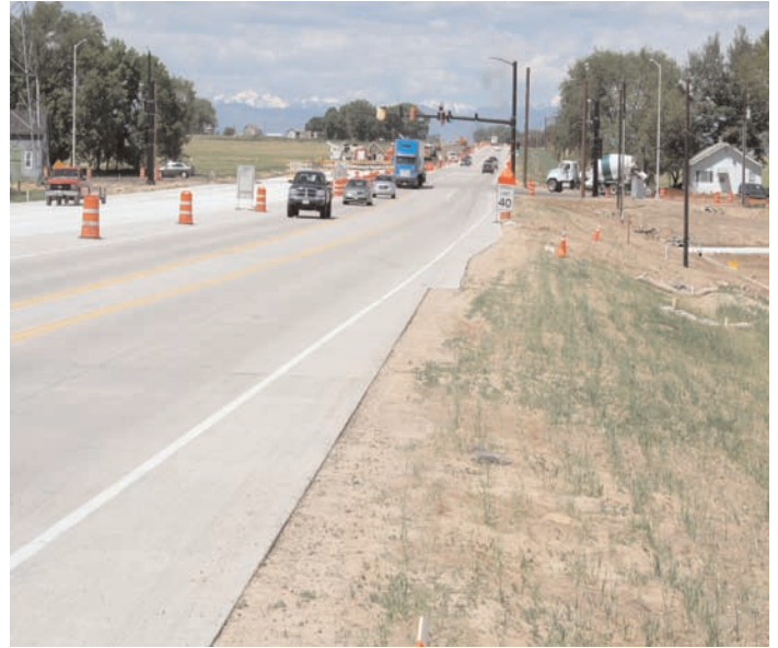
Finished roadway headed West.
