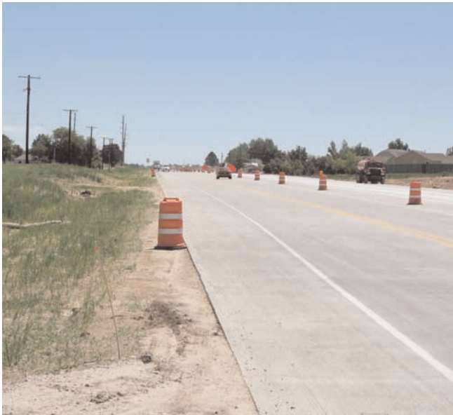
Finished roadway from headed East.
