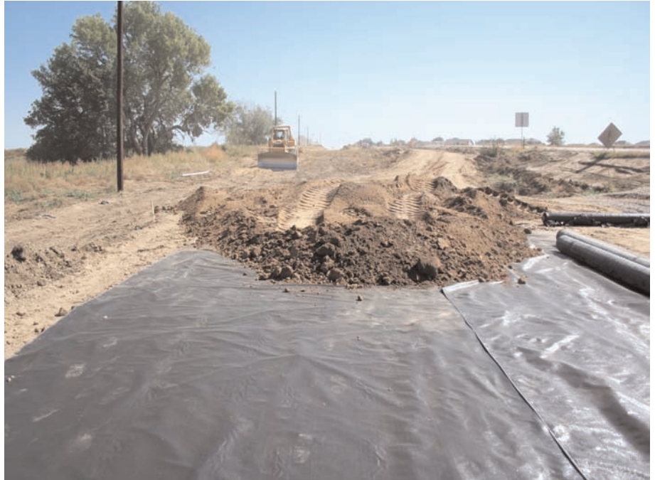
Backfill over Mirafi® HP570.
