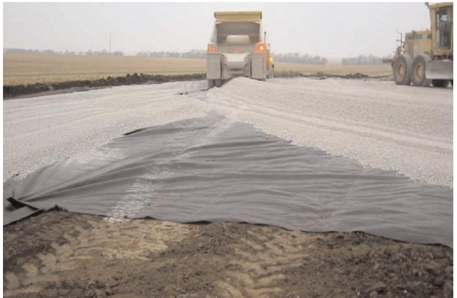
Mirafi® HP570 allows for heavy equipment to drive (while installing crushed limestone) directly on it.
