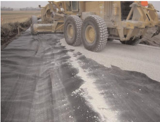
Installing crushed limestone on textile using heavy equipment.
