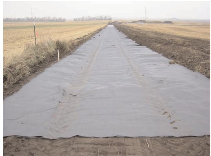
Installing Mirafi® HP570 on soft subbase access road.
