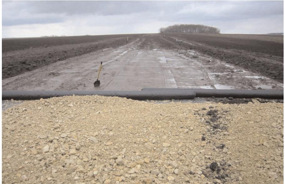
Wet conditions did not stop construction. Mirafi® HP570 separated mud from the crushed limestone.
