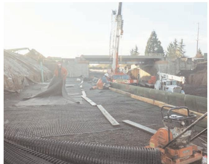
The construction of the MSE walls along the southern portion of the new roadway.
