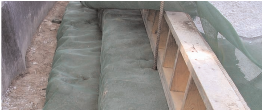
Close-up of temporary form used for the face.
