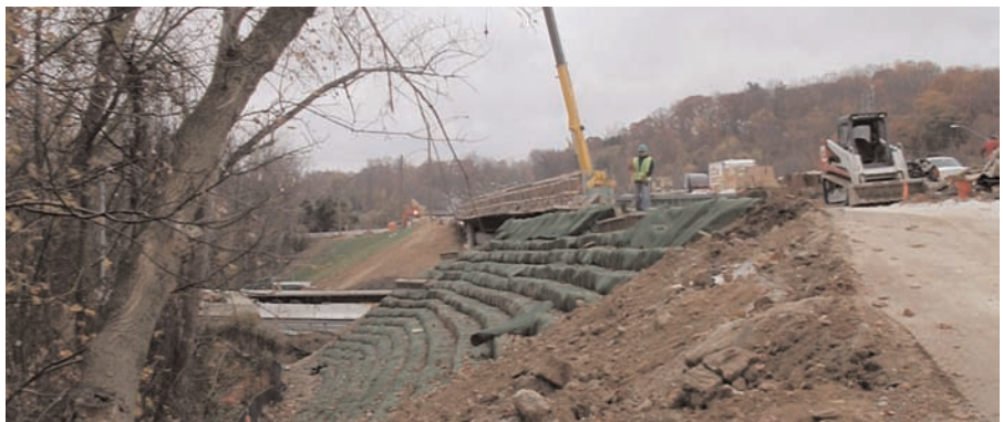
Slope nearing the finished grade.
