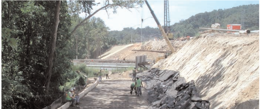
Preparing the drainage fabric behind the slope.
