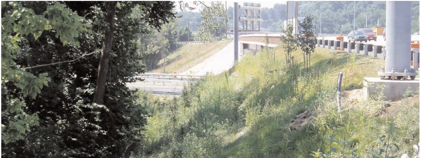
Completed slope with vegetation.
