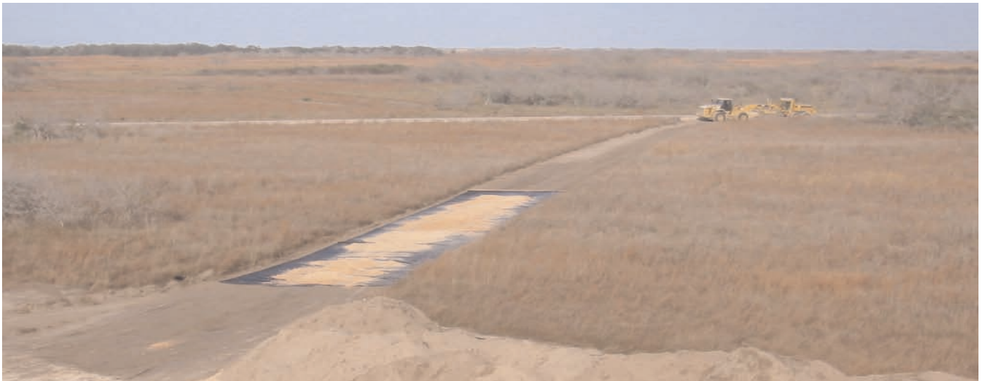
3" to 4" rutting after one pass of construction equipment.
