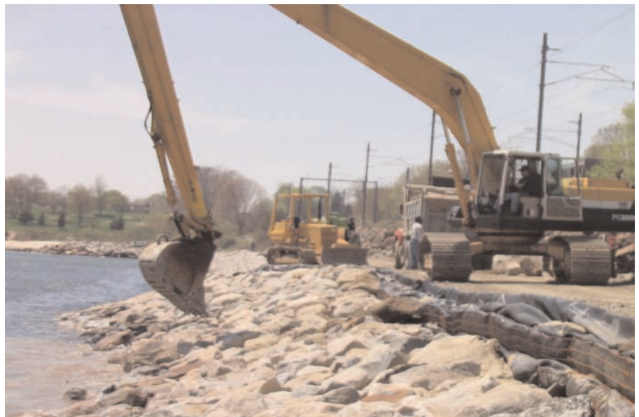
Placing armor stone to protect the Mirafi® FW404 MSE wall.
