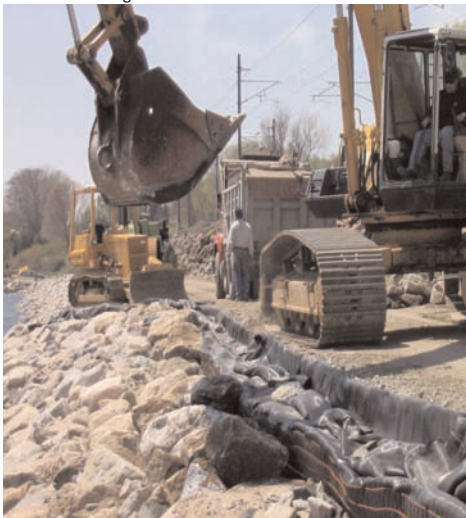
Below: Placing armor stone.
