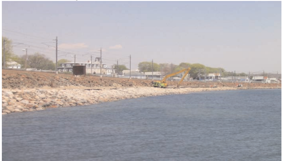
Below: Offshore view during construction.
