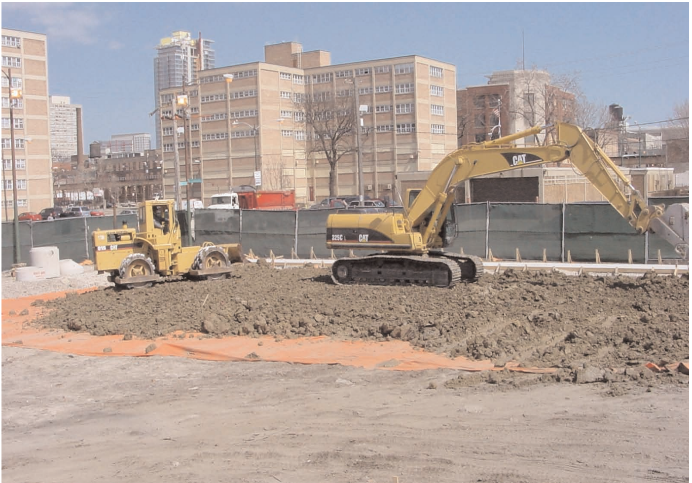
Contractor placing topsoil over Mirafi® Orange delineation fabric.
