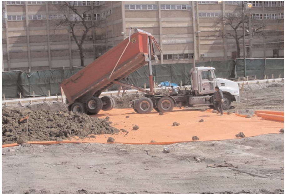
Subsoil condition prior to installation of Mirafi® Orange delineation fabric.
