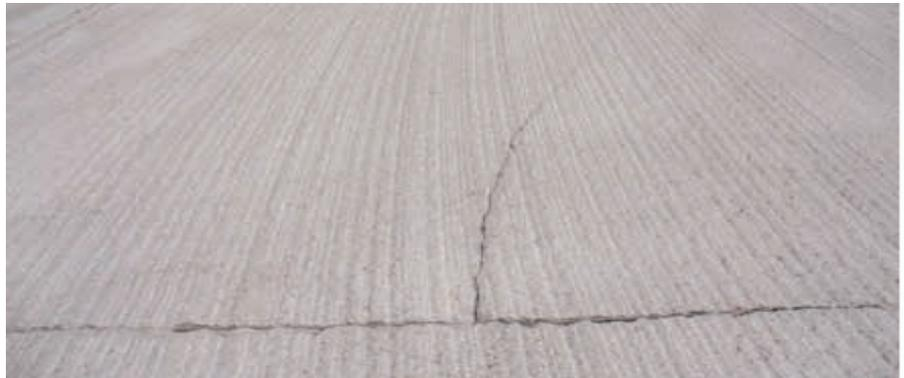
Longitudinal crack and sawed joints in the milled surface.
