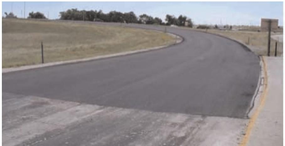
Final surface with Mirafi® FGC100 for tensile reinforcement and moisture protection under 2" of Hot Mix Asphalt.
