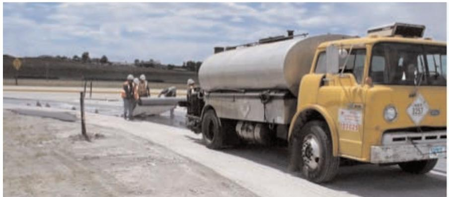
Tack coat is sprayed prior to the placement of the Mirafi® FGC100 to create a moisture barrier to protect the underlying subbase.
