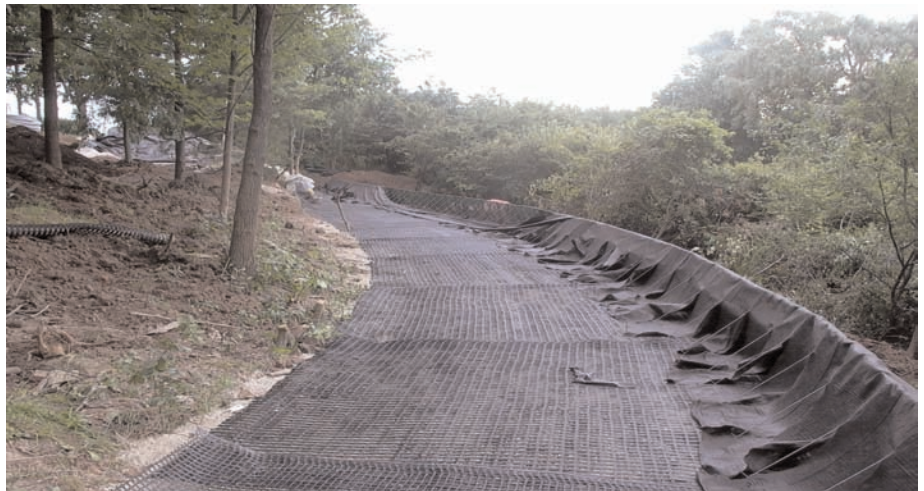
Mirafi® 160N separates the topsoil and granular reinforced zone.
