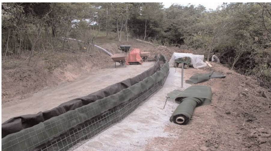
A welded wire wall is constructed with Miragrid® 3XT, Mirafi® 160N, and Miramesh® GR.
