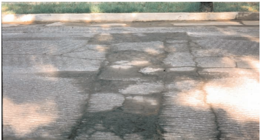
Road after milling, exposing the original cement pavement.
