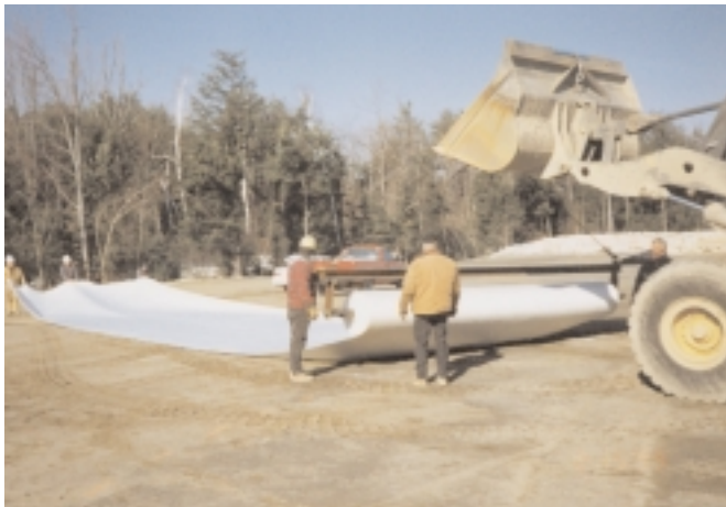
The contractor fabricated a lifting beam and spindle attachment to install the HS4200.
