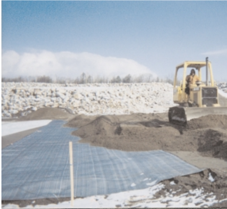
Backfill over the HS4200.
