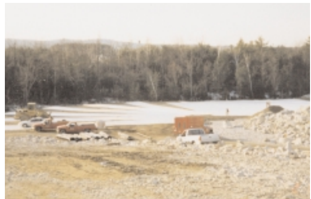
The first layer of HS2400.
