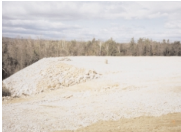
The completed 1:5:1 reinforced embankment.
