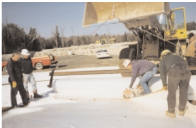
Geolon® HS4200 master rolls were delivered to the job site for efficient coverage.
