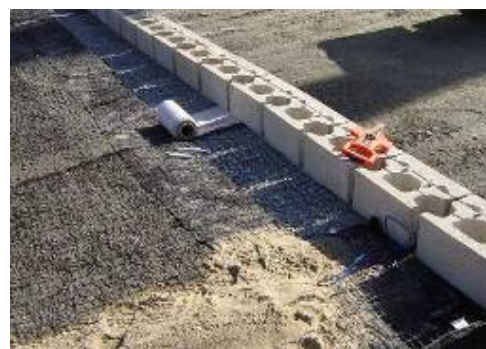
Fig 6(b) 'Intelligent' geosynthetic compliments other soil reinforcement system and providing strain measurements
