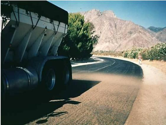
Figure 9: Spreading sand
