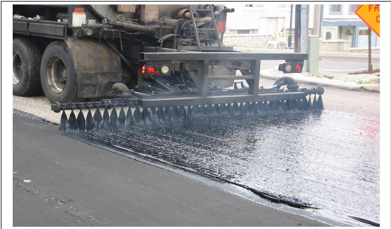
Figure 1: Tack coat being applied
