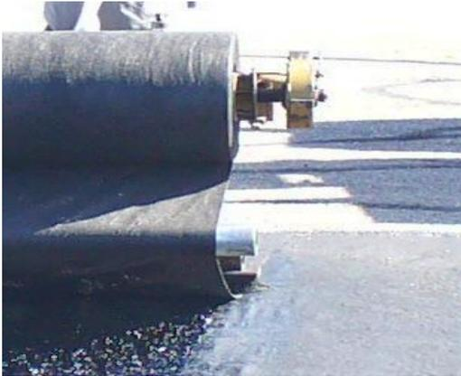
Figure 7: Longitudinal overlap
