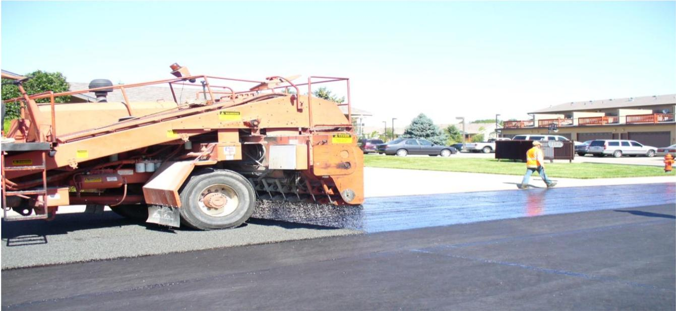
Figure 12: Chip sealing over paving fabric
