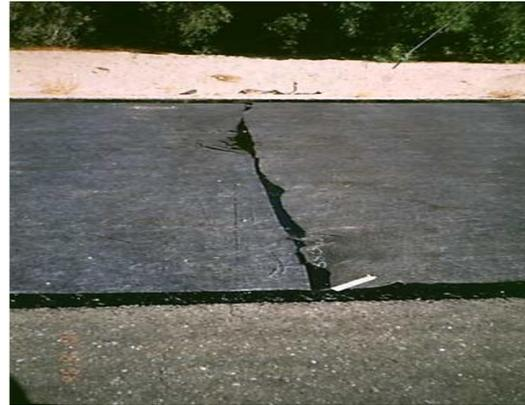
Figure 8: Transverse joint
