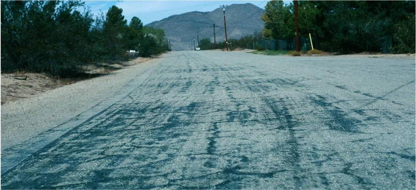
Figure 11: Saturated fabric with sand
