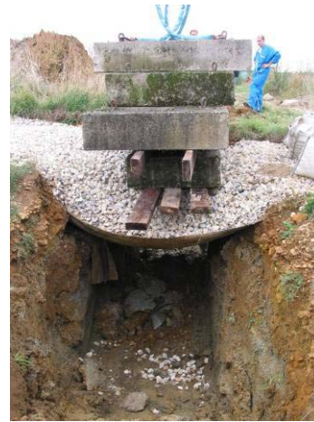
Figure 5(b). Loading test October 2003.
