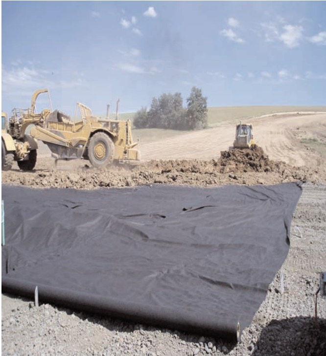
Fill being placed by pan scrapers and bulldozers over the durable Mirafi® 180N.
