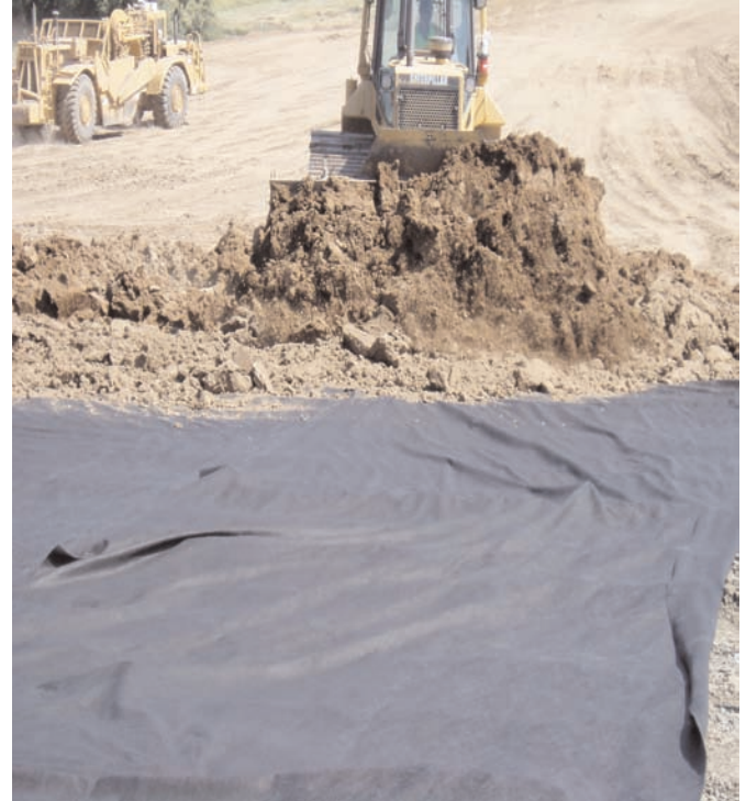
Fill being placed by pan scrapers and bulldozers over the durable Mirafi® 180N.
