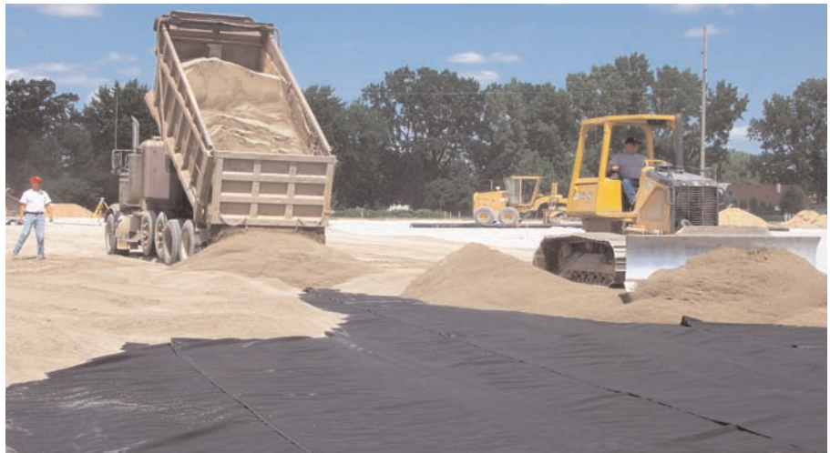
Backfill deployment on Mirafi® FW402 geotextile.
