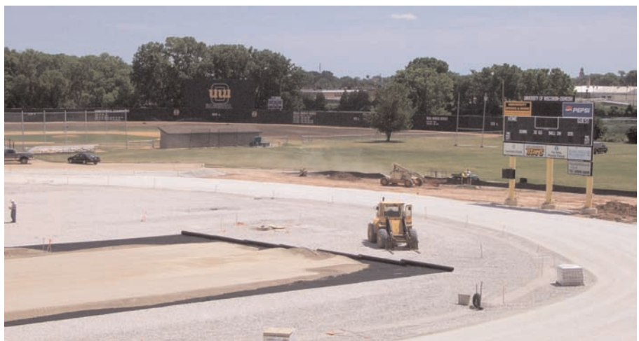
Instillation of Mirafi® FW402 geotextile.
