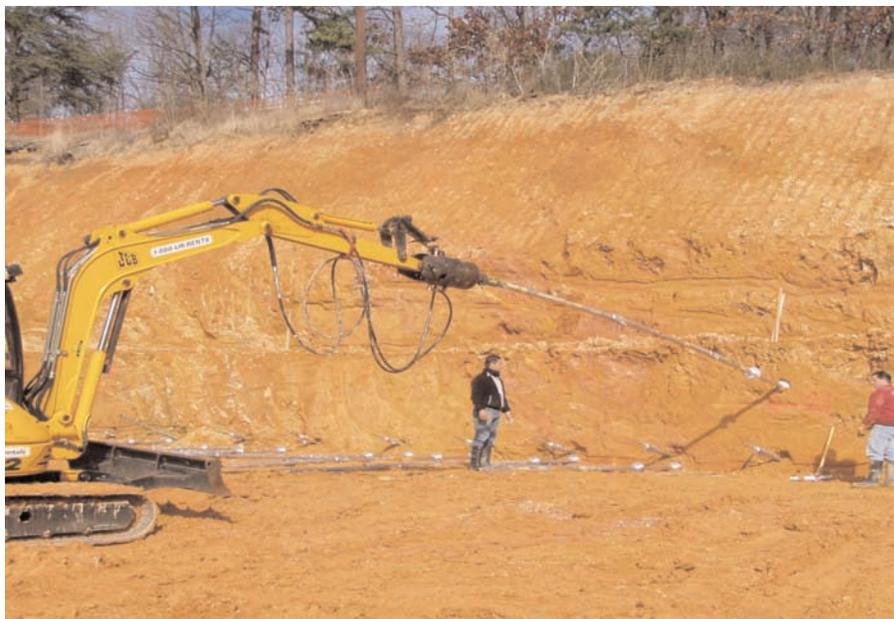
**ABOVE:** Anchor drilling into the side of the cut slope.
