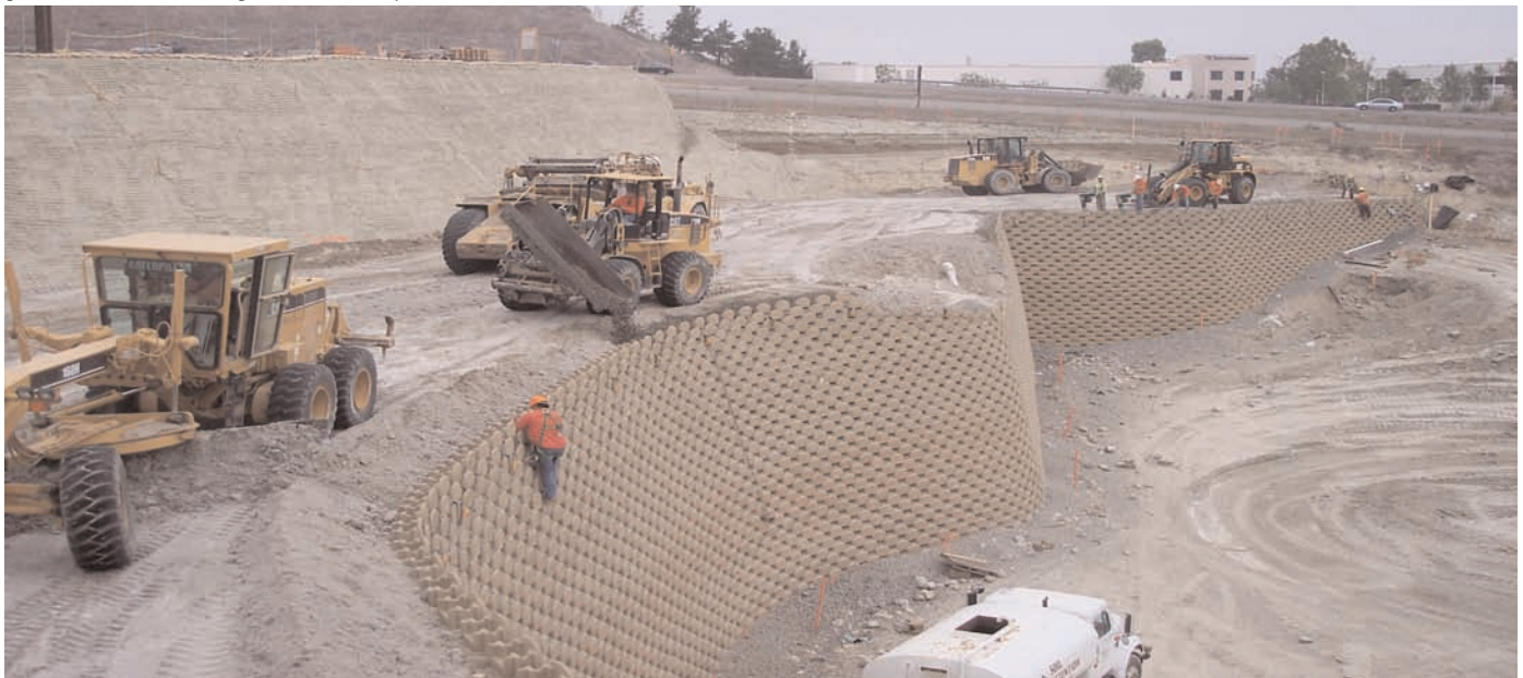
SRS Verdura Wall in construction
