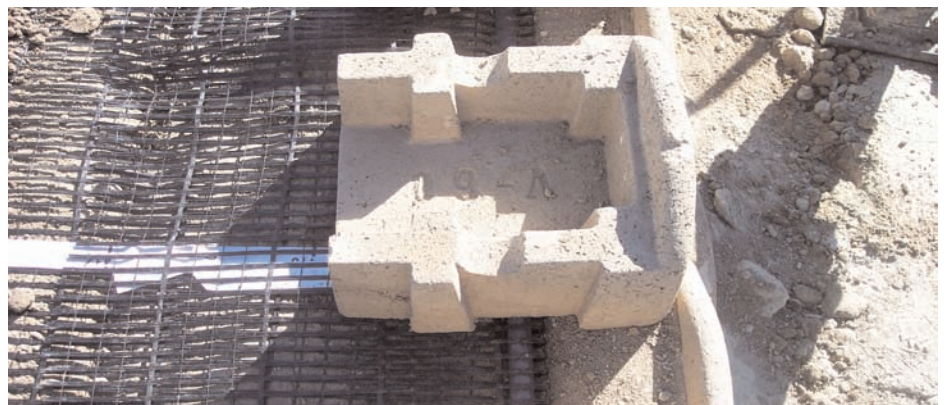
Miragrid® and Schedule 80 PVC pipe connection to Verdura 60 block.
